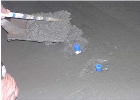
Figure 6.8 – Maturity Meter Installation
