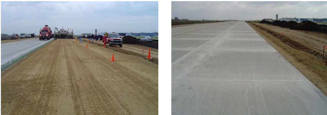
Figure 6.1 - Newly Constructed Taxiway Segment Selected for Field Testing at Aurora Airport
