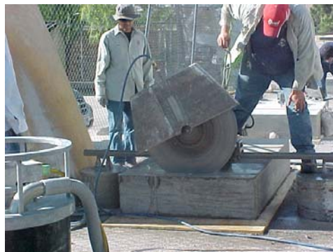
c) Saw-Cutting for Beams
