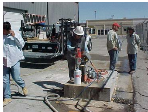
d) Drilling for Cores
